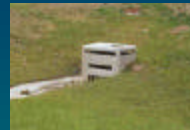
Outflow structure with weirs
